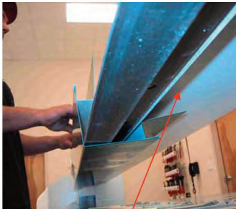
Relief under upper beam
